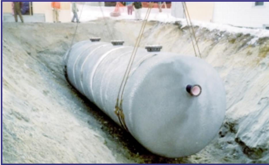
Prestressed Concrete Cylinder Pipe fabricated into a chlorine contact tank, an ideal solution to a common problem.
