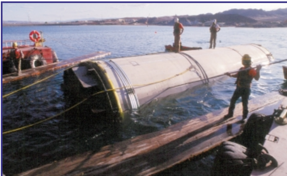
The assembly was positioned in the laying barge.
