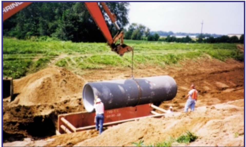
Installation of 60-inch diameter PCCP through trench box.
