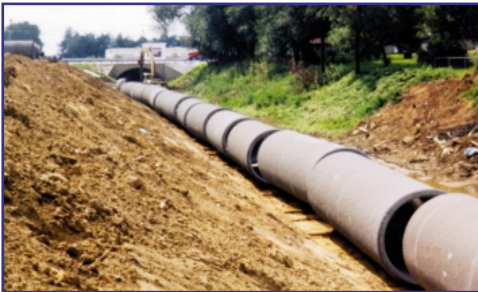
Forty-eight-inch diameter PCCP strung out along the right-of-way, awaiting installation.
